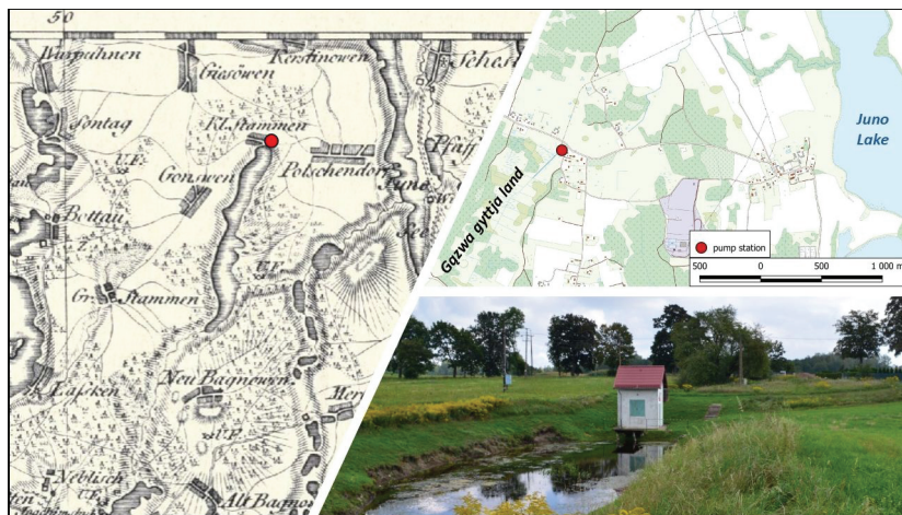
Fig. 2. Water pump station located on gyttja land at Gązwa, NE Poland. Note: the ditch drains water from the former lake, which is then transferred via an underground water pipe to the lower lying Juno lake. The edge of the former lake corresponds to the location of the road. The left map: Stamma lake on the “Map of East Prussia and Prussian Lithuania by F. L. von Schroetter” (1803); the right map: Gązwa gyttja land on contemporary topographic map. Red dot indicates the pump station
